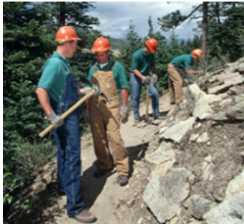
OA trail crew repairing a path at Philmont.
